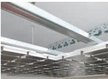
Installation of metal structure with 300 mm pitch
