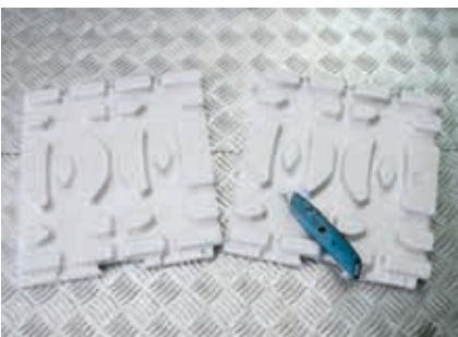
R884 head panels cut to measure
